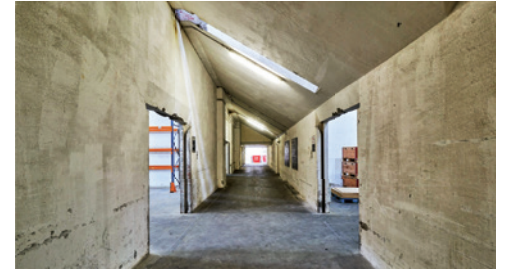
Anciens silos © Martin Zeiler
